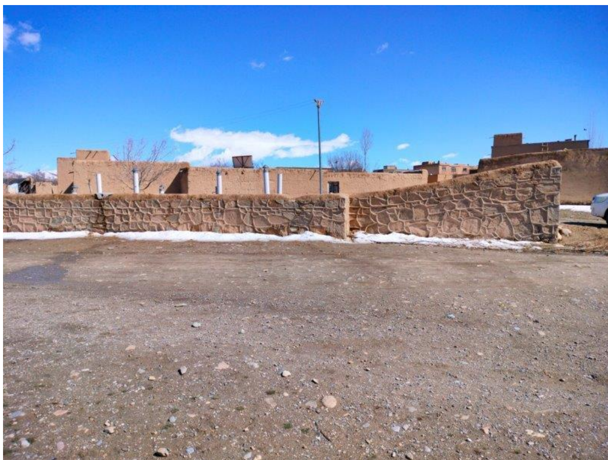
PICTURE 1 – SIDE ELEVATION OF POTATO COLD STORAGE IN BILCHERAGH DISTRICT CENTER
