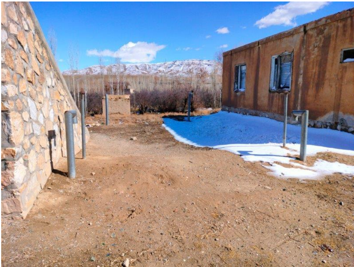
PICTURE 9 - POTATO STORAGE, QUSH VILLAGE, GHAZNI CENTER (VENTILATION)
